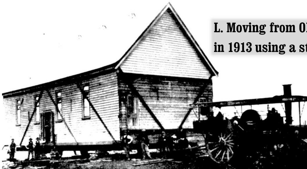
**L. Moving from Old Cororooke in 1913 using a steam engine.**
